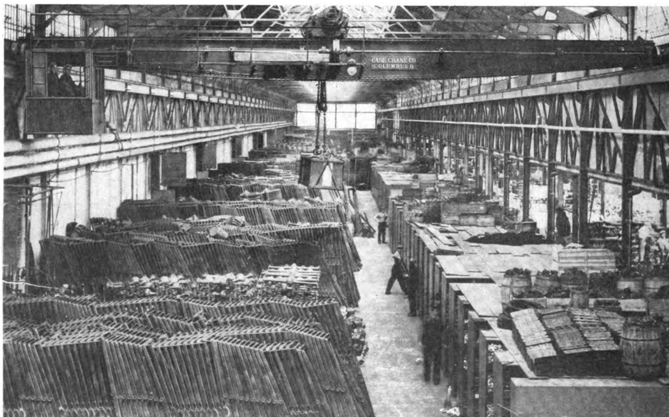
Giant crane which runs the length of the frame arm of the factory. The crane spans that section of the factory and has a track 800 feet in length
